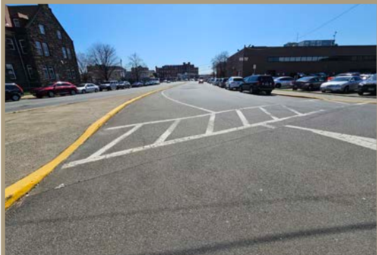
Figure 16. Looking south at the very wide right turn lane onto State Street.
