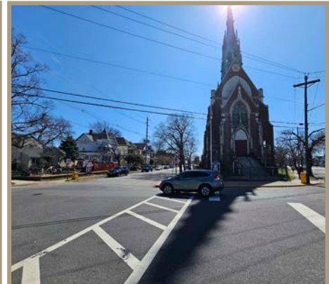
Figure 26. Looking south on Hamilton, a vehicle blocks the crosswalk to see traffic.
