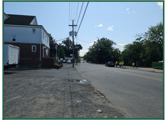
Figure 19. Missing sidewalk on east side.
