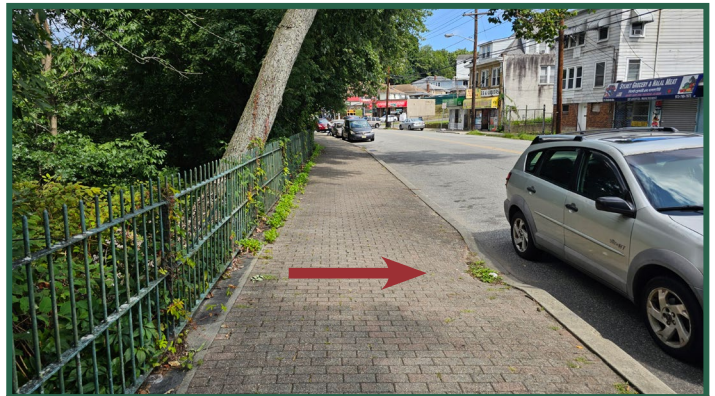
Figure 26. Non-compliant curb ramp blocked by parked car.
