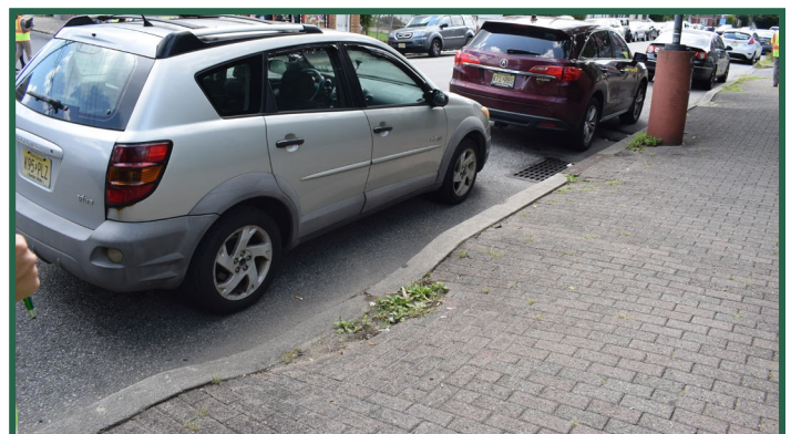
Figure 48. Blocked curb ramps.
