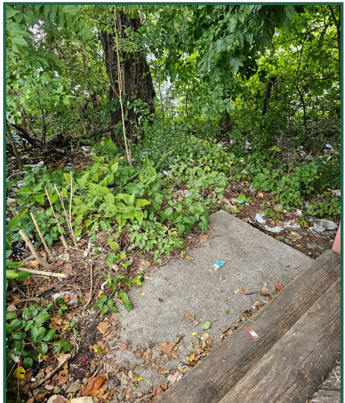
Figure 37. Stairs with unclear purpose leading down to river have collected litter.
