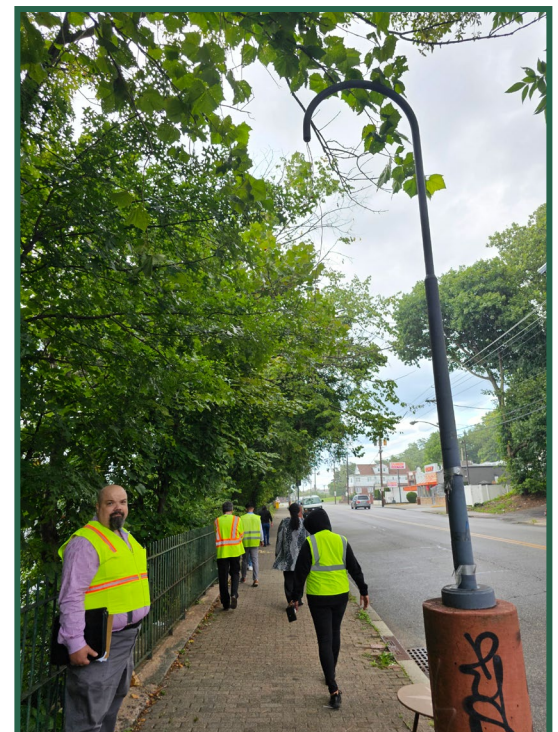
Figure 27. Vandalized light fixture.
