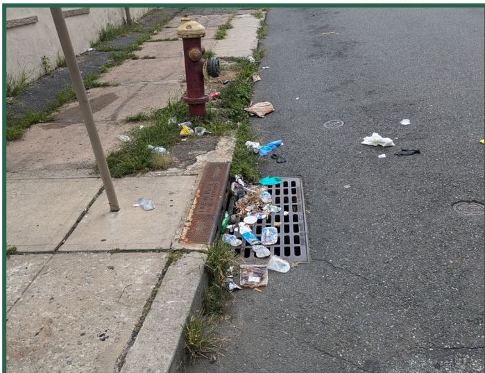
Figure 32. Trash on storm drain.
