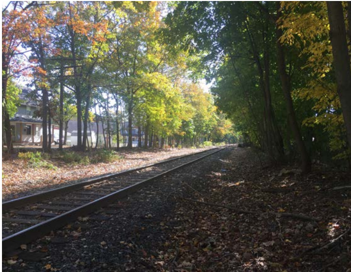
FIGURE 107. PEDESTRIAN AND BICYCLE RAIL CROSSING LOCATION
