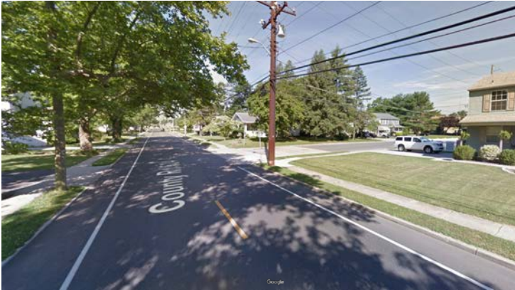
FIGURE 86. STREETVIEW E HOLLY AVE & CLINTON AVE
