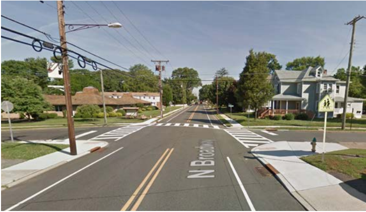
FIGURE 26. EXISTING N BROADWAY AND WOODLAND AVE
