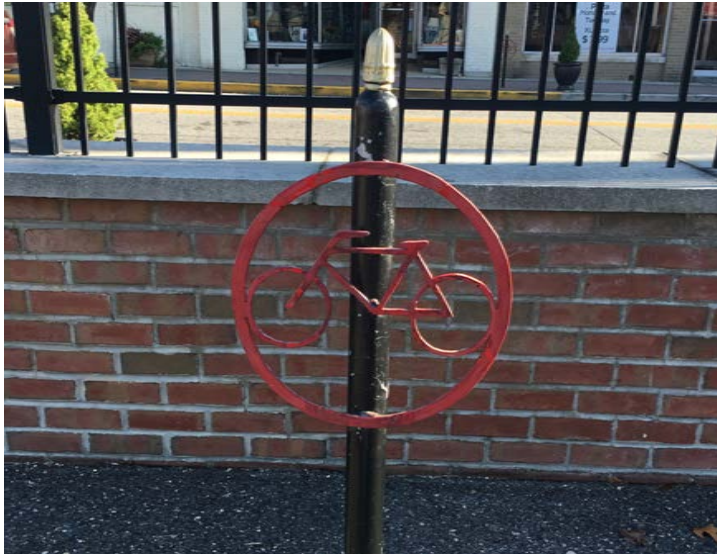
FIGURE 145. POST AND RING BICYCLE RACK NEAR BROADWAY AND HOLLY AVE
