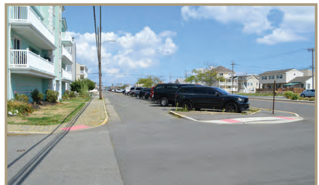
Figure 22. Missing "Do Not Enter" sign on service road.
