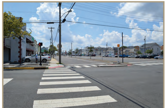
Figure 41. Looking south from Grant Avenue, a curb extension creates a mandatory right turn.
