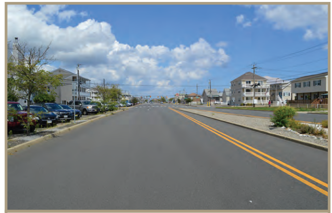
Figure 32. Looking north at lane merge.
