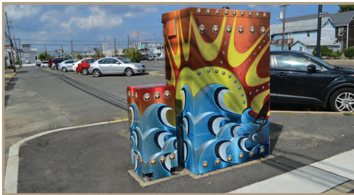
Figure 25. Traffic signal control boxes wrapped with art.
