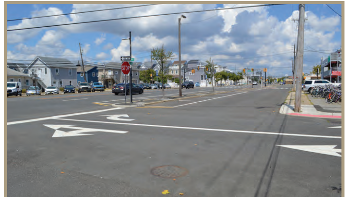
Figure 16. Confusing intersection with service road.
