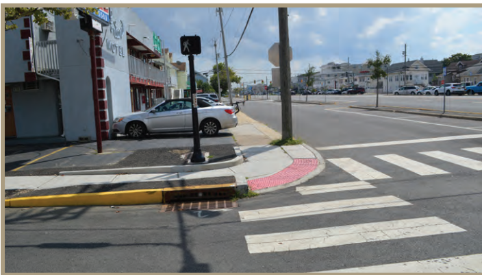
Figure 17. ADA compliant curb ramps.
