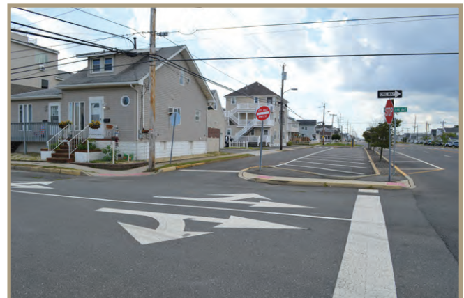
Figure 34. Stop bar beyond the frontage road.
