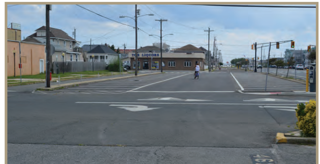
Figure 21. Missing signage makes traffic direction on service roads unclear.
