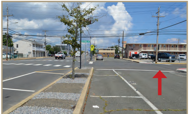
Figure 43. Incomplete crosswalk seen at Sherman Avenue in background. In foreground, missing trees.
