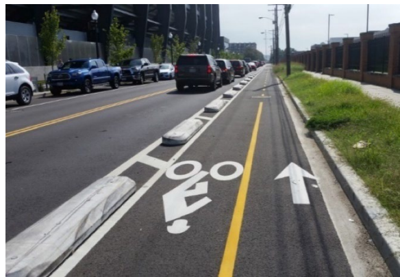
Figure 5: A curb-protected two-way bike lane in Washington, DC (Photo: Stephen Hudson in Alpert, 2019)
