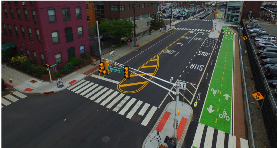
Figure 7: A two-way protected bike-lane with flexible plastic bollards on Observer Highway in Hoboken, NJ (City of Hoboken, NJ, n.d.)
