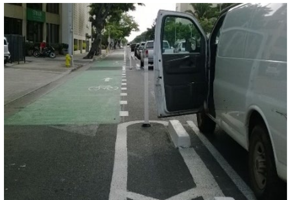
Figure 6: The buffered door-zone of a curb-protected one-way bike lane with parallel parking in Honolulu, HI (City & County of Honolulu, 2018)
