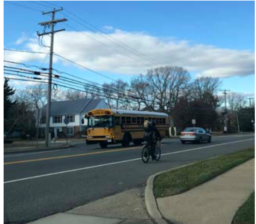
Example of typical County road - Old Freehold Road
