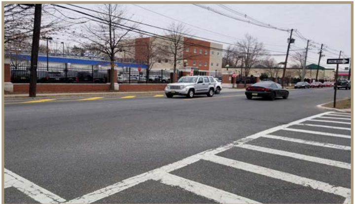
Figure 19. To the right of the intersection, a crosswalk is missing over North Avenue.
