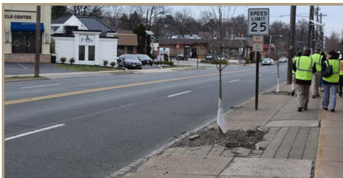
Figure 15. Cracked and uneven sidewalks and pavers, looking eastward on North Avenue near Central Avenue.
