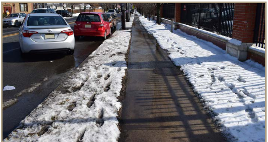
Figure 64. Flooding along the sidewalk, looking eastward near the intersection of St. Paul Street and North Avenue.
