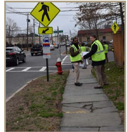
Figure 14. Cracked and raised slate sidewalks, looking westward at the intersection of St. Paul Street and North Avenue.
