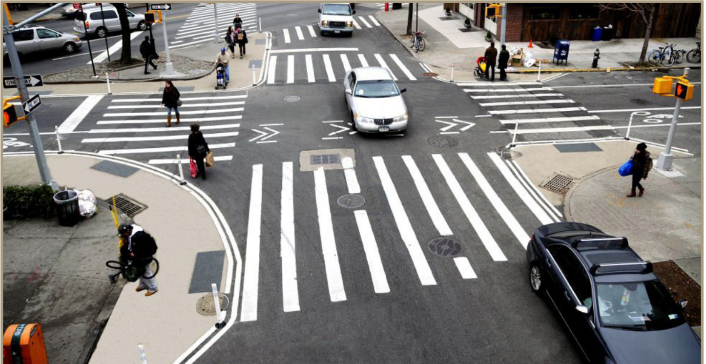
Figure 63. New York City has made extensive use of paint and plastic bollards to decrease turn radii at intersections throughout the city.
