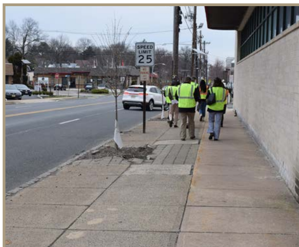
Figure 33. No barrier between pedestrians and large volumes of traffic, looking eastward on North Avenue near Central Avenue.
