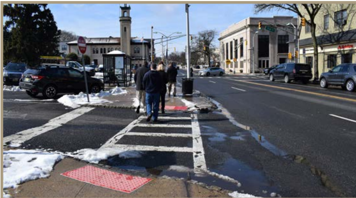
Figure 20. Misaligned accessibility ramp with drainage issues, looking westward at the train station entrance (photo taken during initial site visit).
