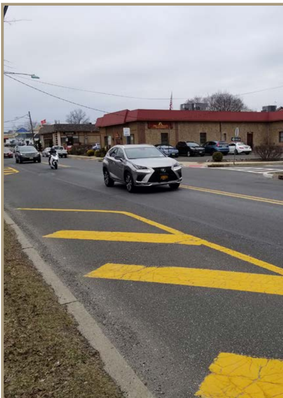
Figure 66. Location along North Avenue where second travel lane abruptly ends (looking west on North Avenue).
