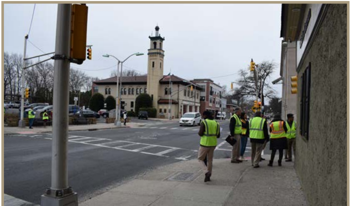
Figure 21. Pedestrian signal heads are missing at the intersection of Elm Street and North Avenue.
