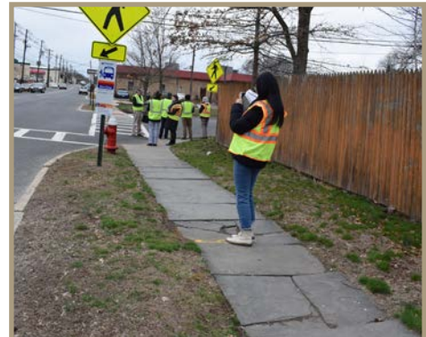
Figure 30. Cracked slate sidewalks near St. Paul Street, looking westward on North Avenue.
